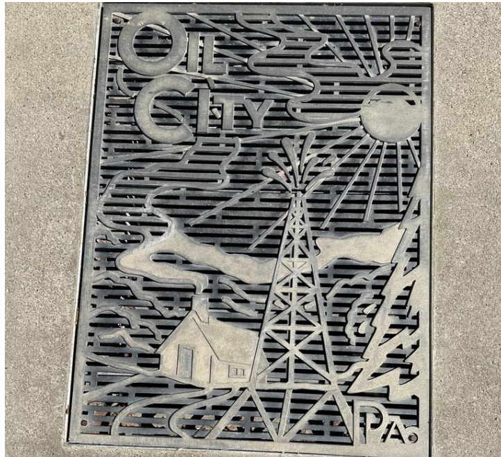
Figure 8. A Storm Drain in Oil City, PA
